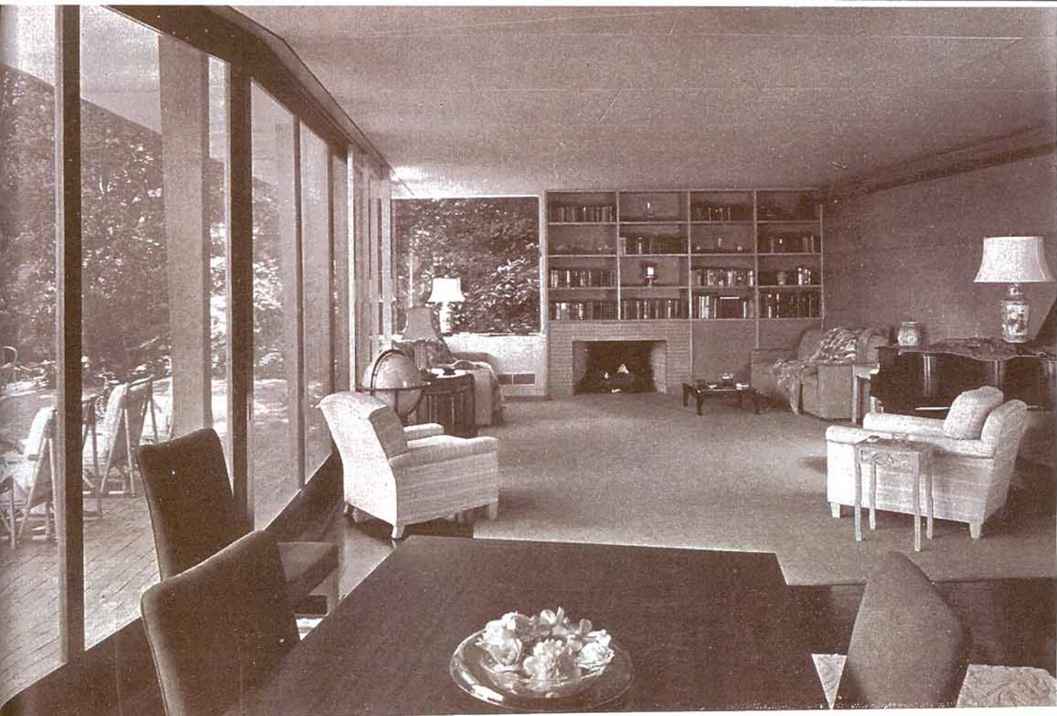
STANDING WOODEN POSTS CARRY LOAD OF LIVING-DINING ROOM ROOF INDEPENDENTLY OF SOUTH WALLS, COMPOSED ENTIRELY OF GLASS
