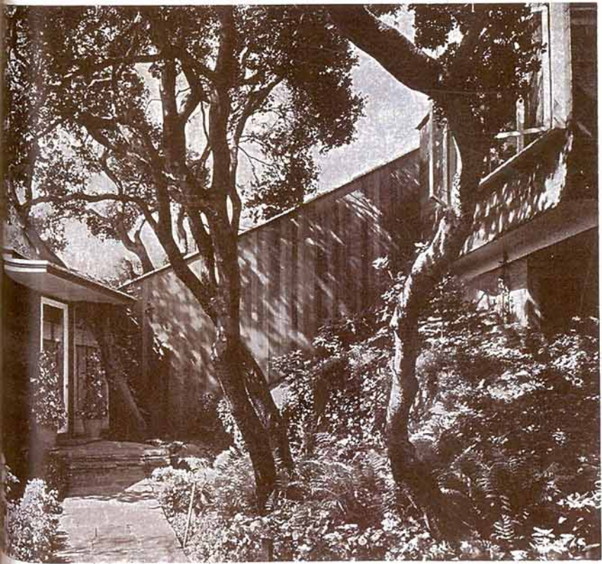
ENTRANCE IS LOCATED NEAR CENTER OF HOUSE AT LOWER END OF STAIR-PASSAGE
